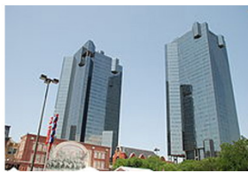
City Center towers Fort Worth Texas Provided: vibration / noise control
