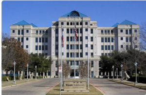
Cooks Childrens Fort Worth Texas Provided: vibration / noise control
